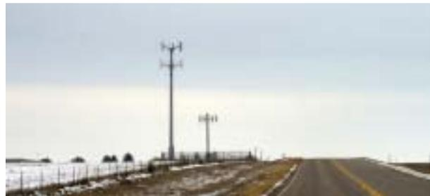
*Figure 36—Wireless communication towers are highly visible in more open areas of the Corridor and should be integrated with existing structures whenever possible.*
